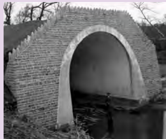
Wingohocking sewer outlet. Source: Department of Records, 1929
